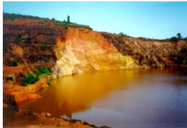
Pit slope failure in a surface iron mine of the Goa district - India
